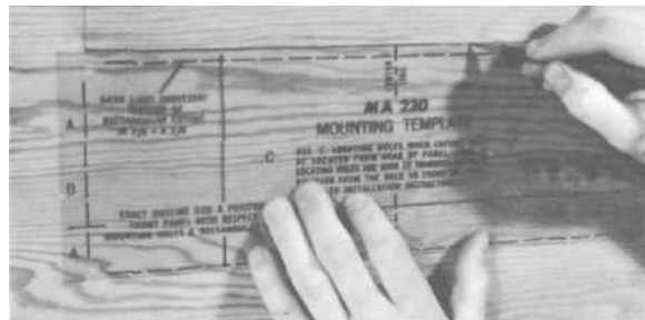
Figure 18. Marking the Cutout Indications.
